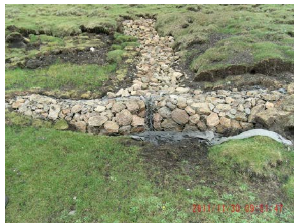
Sack Gabion and Rock Pack
