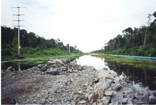
Fig. 2.1c : “Displacement Method” of Road Construction on Peat & Organic Soils along Salim/New Airport By Pass
