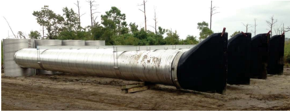
Figure 5: Water control structures at Alligator River NWR ready for installation. Tide-check flex valves installed on the outlet end to prevent saltwater intrusion upstream of water control structures. Photo courtesy of TNC.
