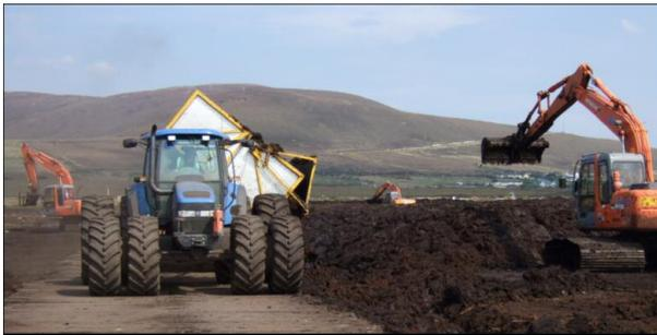
**Figure 5.** Peat being discharged and placed in final deposition area.
