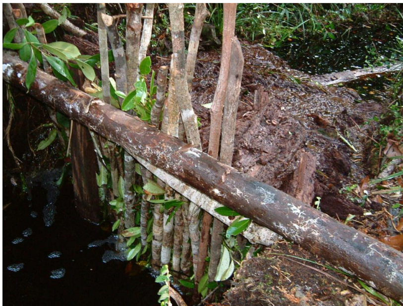
Figure 2. Dam in illegal logging canal in the Sabangau catchment, Central Kalimantan, Indonesia, constructed using local available material.
